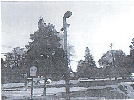
Image 6 – Pole Lighting with Floods
